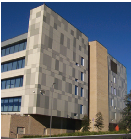
Woolworths Corporation Centre, New South Wales
