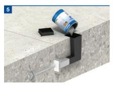
Mix the two-part epoxy resin and pour into the void former. It is essential the resin flows along the stainless steel box section towards the joint and reaches the notches on the locking plate, which indicate minimum resin depth.
