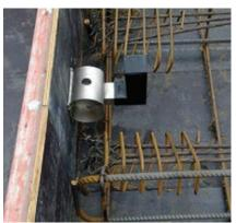
HLDQ-L30 Sleeve nailed to formwork
