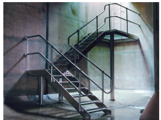
Access Walkways and Ladders
