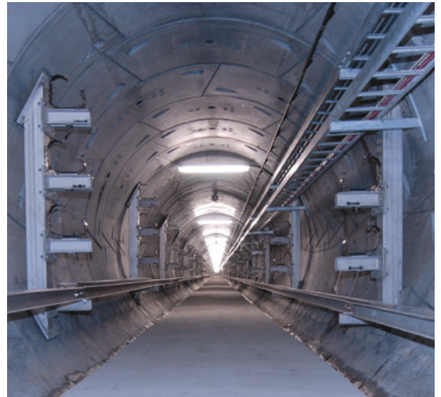
Project: City West Cable Tunnel, Australia (Client: Energy Australia, Contractor: Thiess, Engineer: Maunsell/AEcom)
