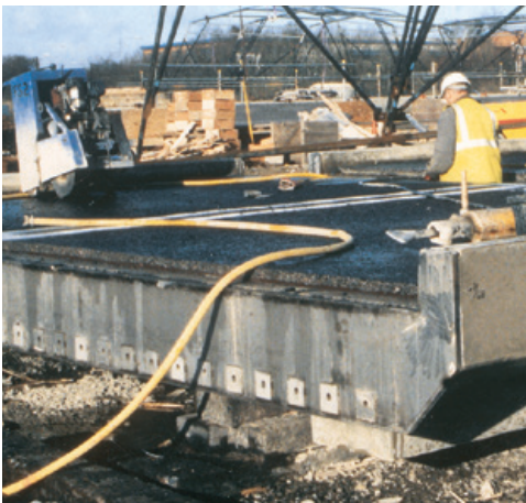
Road Deck Endplates. Project: Dartford East Tunnel, UK (Contractor: Kvaerner/Skanska)
