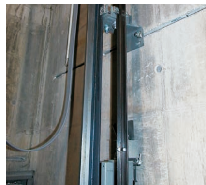
Elevator Guide Rail Connected By Anchor Channel
