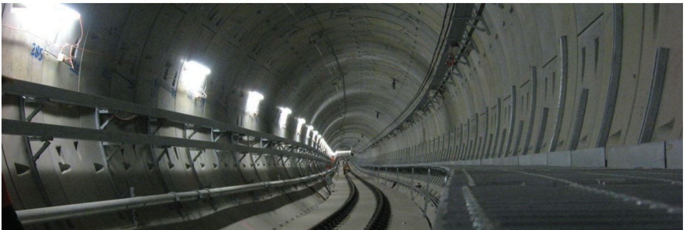
Steel Walkway, Perth MetroRail City Tunnel, Australia
