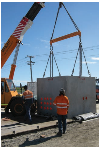
R8 hanger bar with hooks for 1.3t RA anchors
