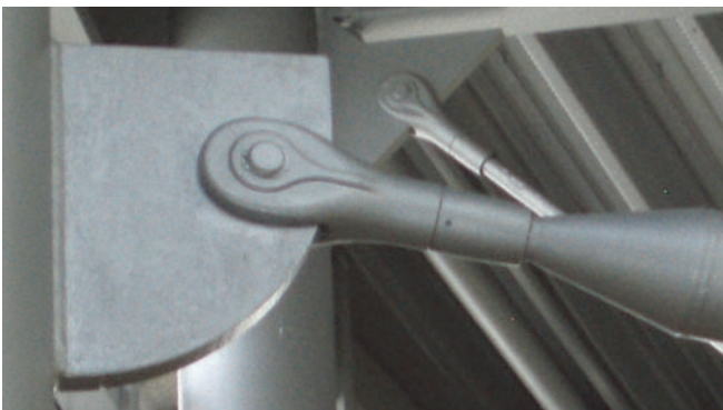
Compression system connected to a welded plate
