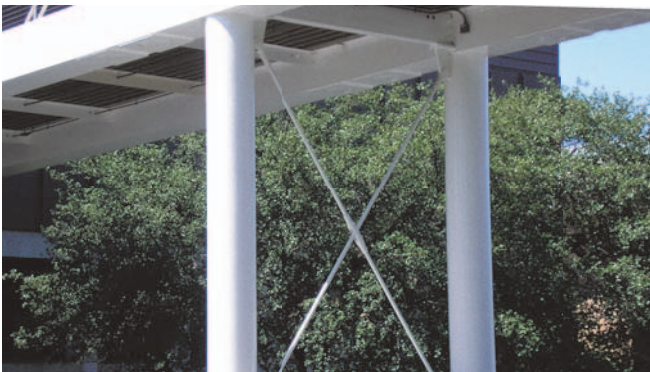
Cross-bracing with a cross coupler
