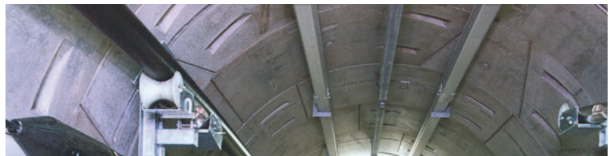
Curved Halfen Cast-in Channels in tunnel segments
