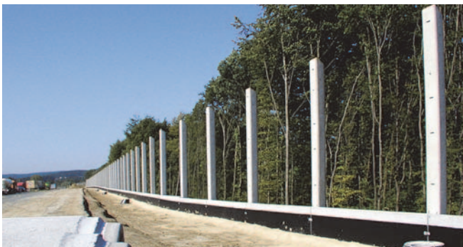
Fixings of noise barriers to concrete posts
