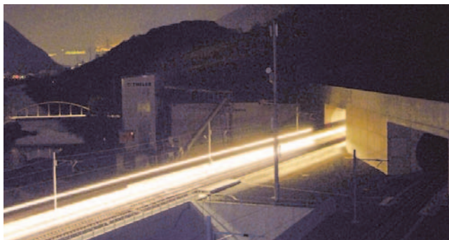
Lötschberg-Base tunnel, Switzerland
