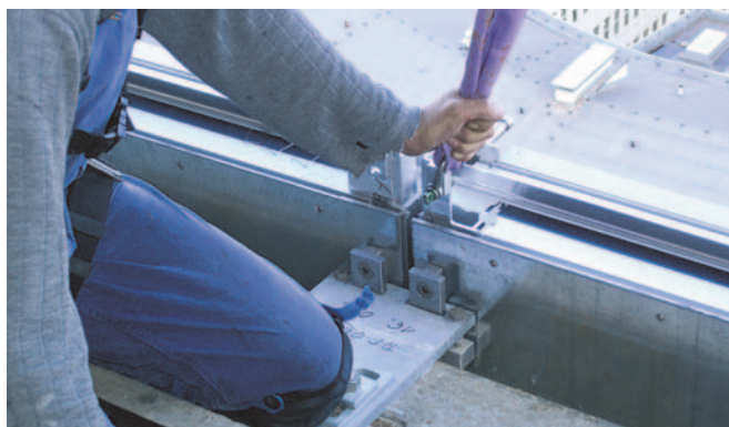
Fixing of a modular façade using HCW-ED Brackets on HTA-CE Cast-in Channels
