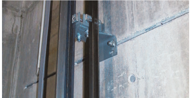
Fixing guide-rails with Halfen Anchor Channels
