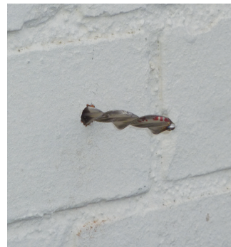
1. Install tie into inner or outer leaf masonry.
