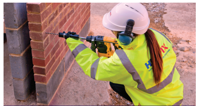
DryFix tie being power-driven into pilot hole
